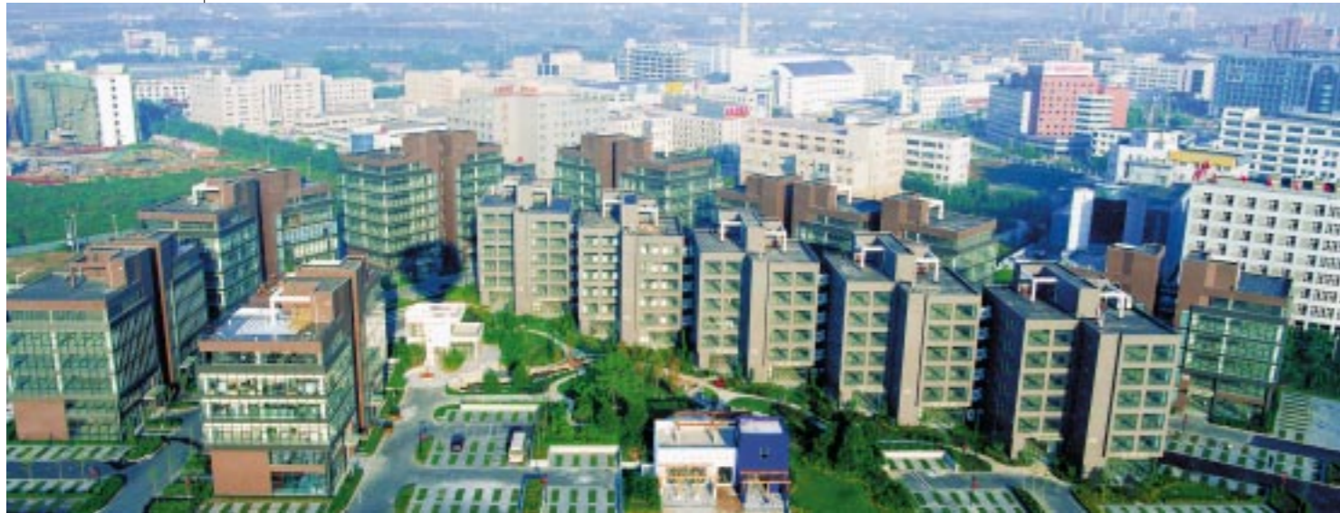
One corner of the 65-hectare, 500-building ABP development.
