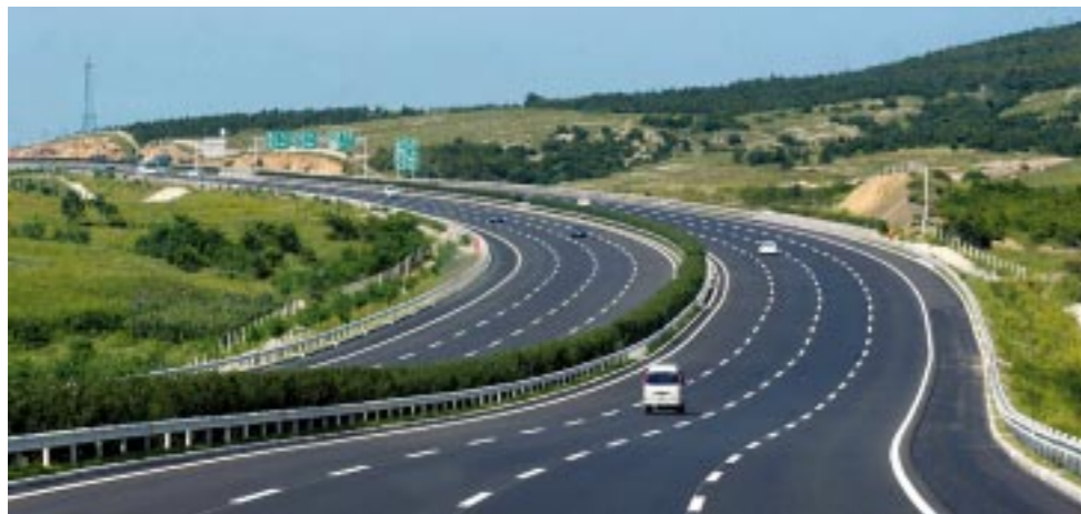
Feeding the “1 line,” the $901-million Shenyang-Dalian Expressway. by China Foto Press
